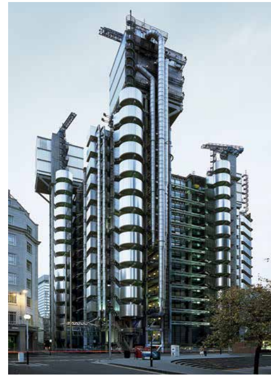
Lloyd's building. R. Rogers. 1986.
